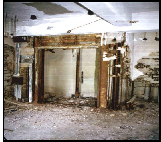
(Otis) elevator shaft, Note all of the misc. water pipes, power, and air ducts.
