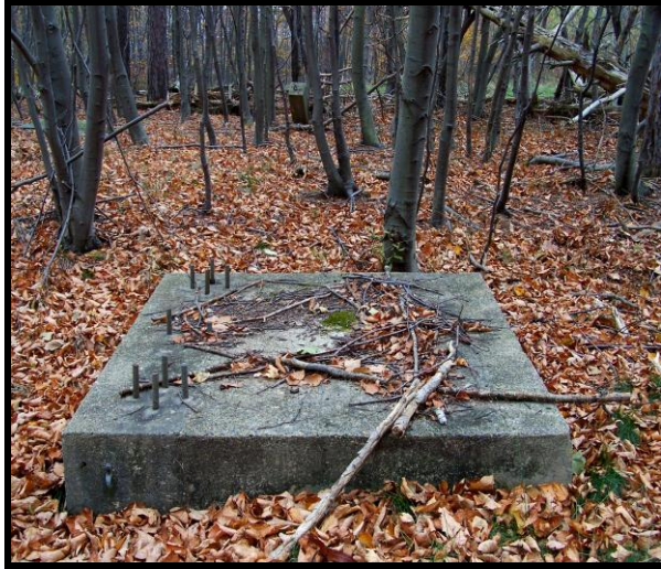
Base of the LP Antenna and Anchor for one of the Guy Wires
