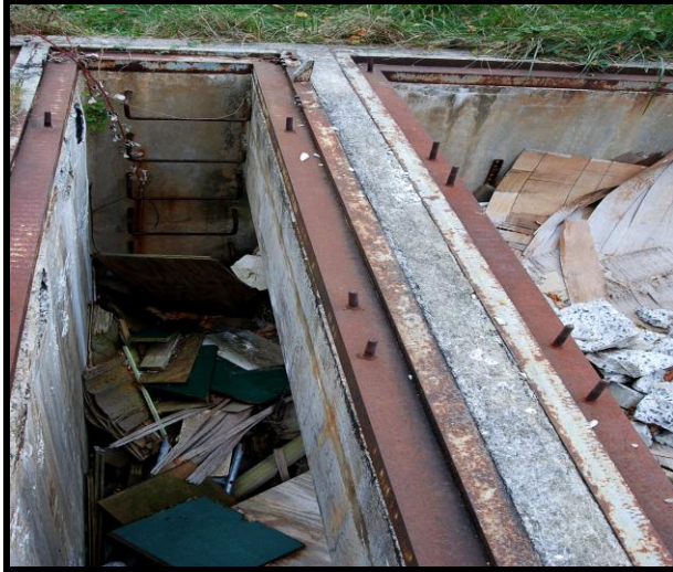
The generator pit filled with debris
