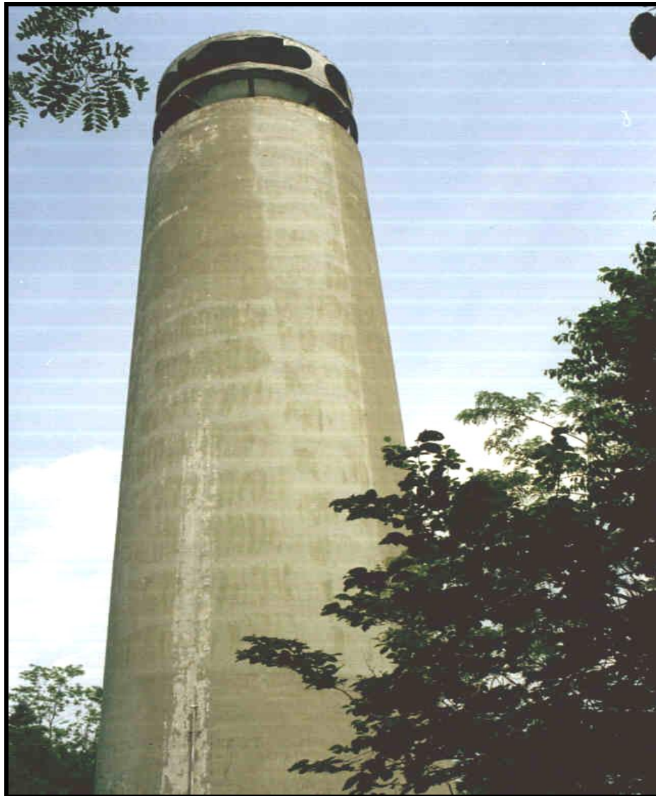
103' tower, "The broken Plexiglas layer at the top is quite visible. A sharp piece falling from the top could kill!"
