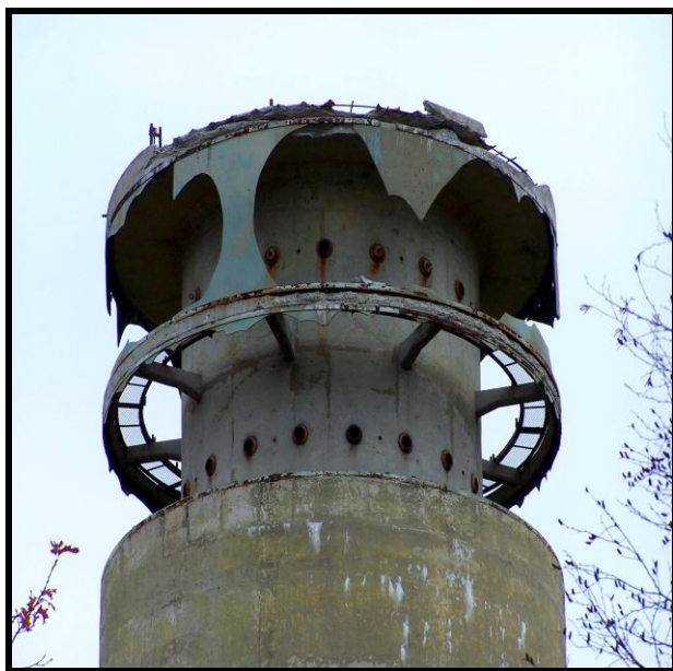
The top two floors were the antenna decks originally enclosed by Plexiglas
