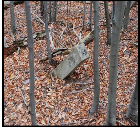
Base of the LP Antenna and Anchor for one of the Guy Wires
