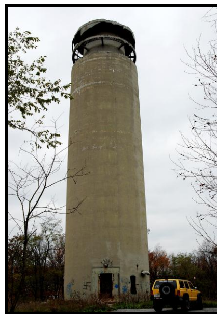
The top two floors were the antenna decks originally enclosed by Plexiglas
