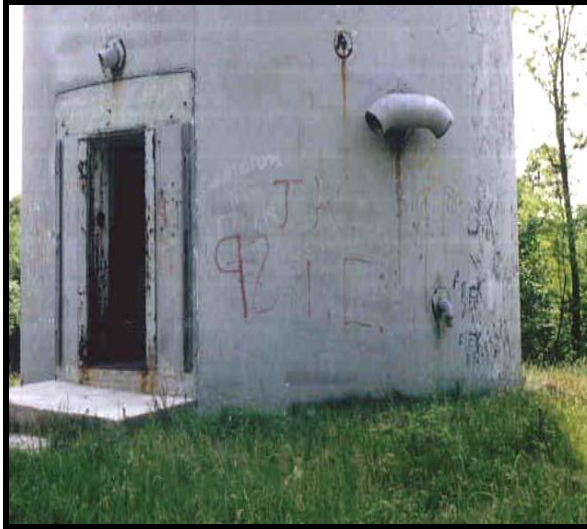
Sole entrance/exit (blast door is missing) in 1999, steel plate covers entrance in 2011
